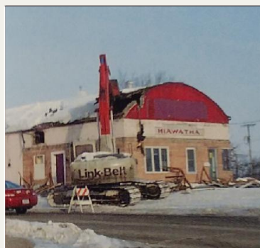
Quonset Building Demolition March 2008
