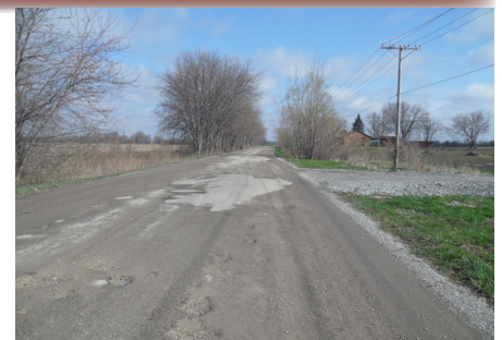
Stamy Road Project
