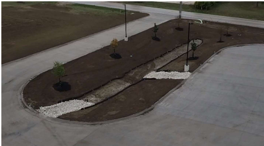
Buresh Construction Detention Basin
