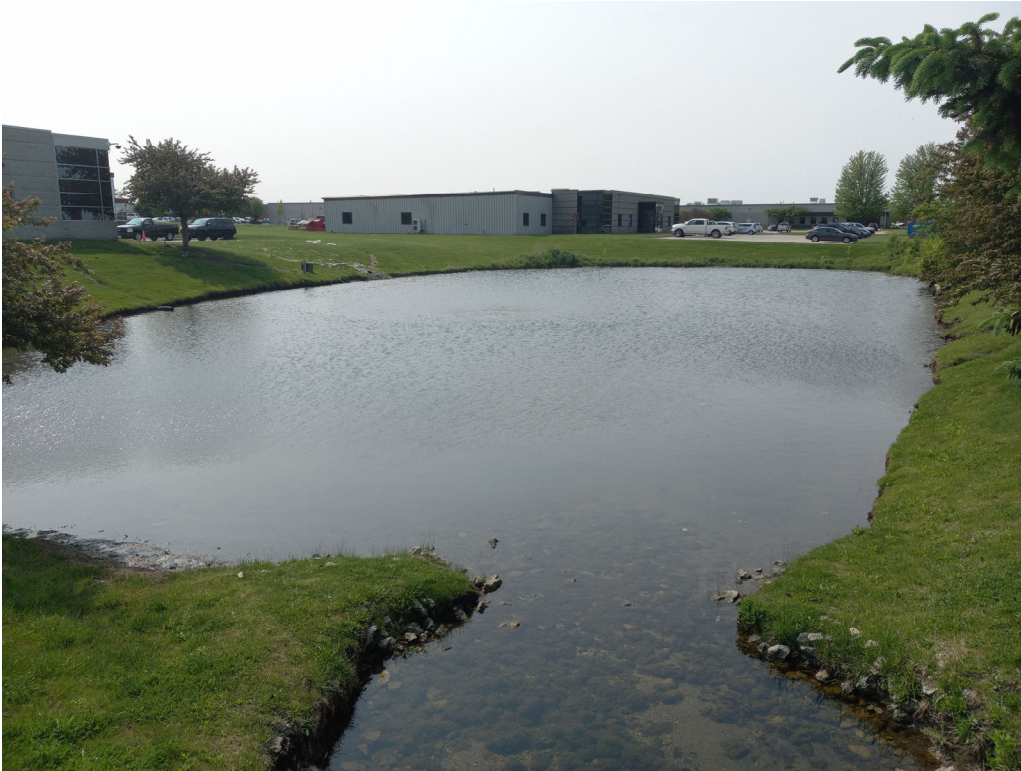
Photo #1: View of the detention basin standing at the northwest corner and looking south. The forebay for the storm sewer discharging into the basin that is shown in Photo #2 is in the foreground of this picture.
