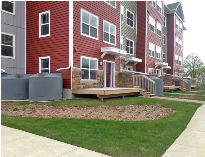
Above ground rainwater harvesting cisterns in Cedar Rapids capture water to be used for gardening and irrigation.
