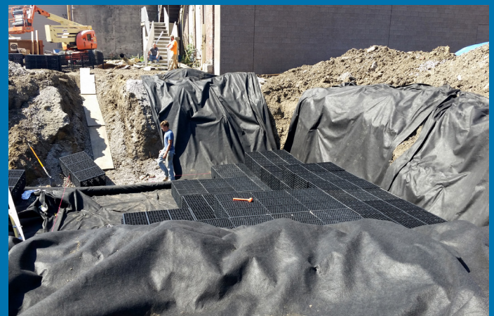
These structural blocks and plastic liner are used to store water below ground. They are used as the reservoir below natural or landscaped water features, like shown above and on the front page.
