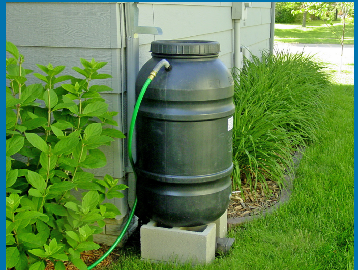
Rain barrel capturing rainfall from homeowner's roof to be used for watering plants.
