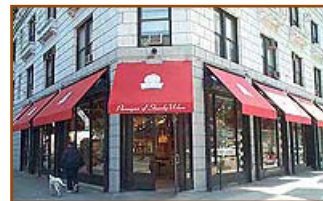
A good example of mounted awnings placed below the horizontal expression line.
