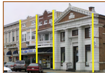
Desired vertically-proportioned buildings.
