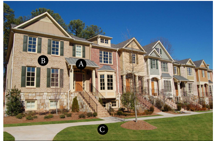
This graphic illustrates how a row house can use varying techniques to create a relationship with the street (See text for technique descriptions)
