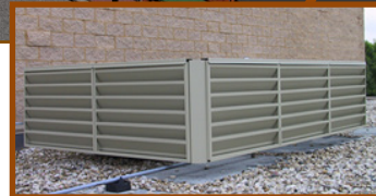
Example of a building facade screening rooftop mechanical from ground view.
