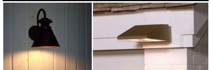
The upper graphic illustrates the different types of lighting techniques from no cutoff to full-cutoff. The lower images provide good examples of full-cutoff building light fixture
