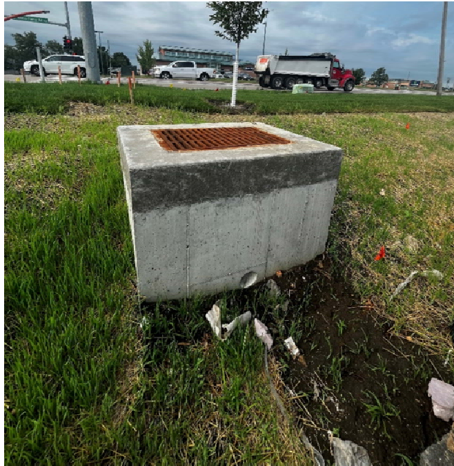
Photo 4: View of the Completed South Detention Basin Outlet Structure
