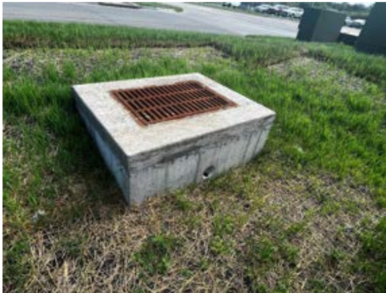
Photo 1: View of Completed North Detention Basin Outlet Structure
