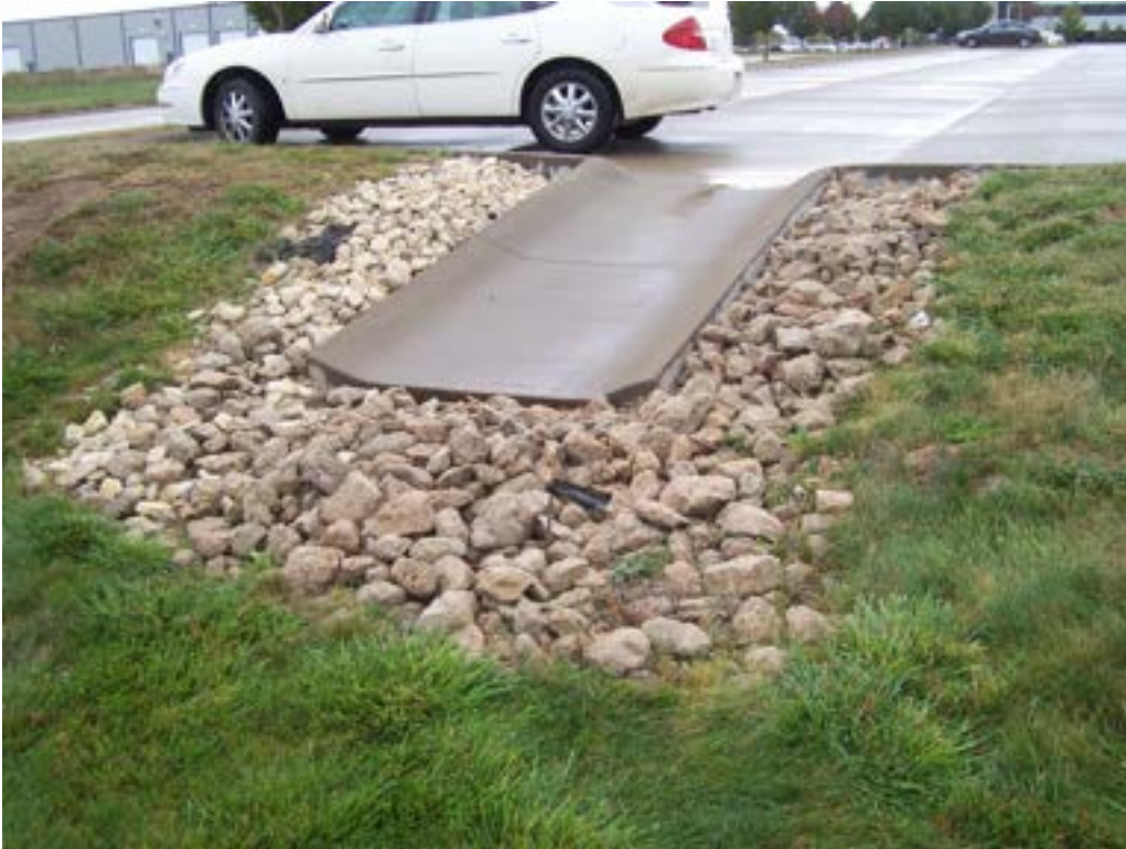
Photo #2: View of drainage flume discharging into the east end of the detention basin.
